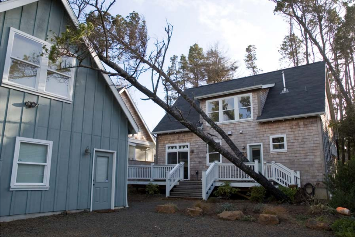
Some of the December 2006 storm damage at Bella Beach...
